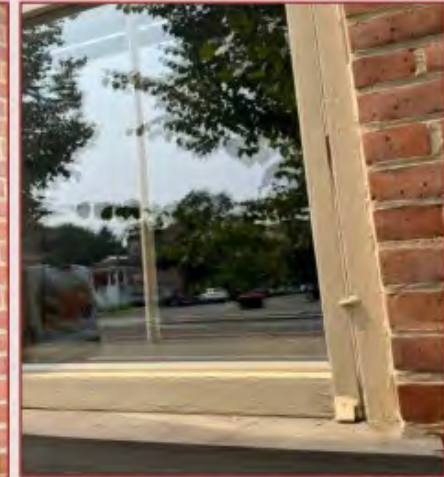
Above: 2 Broad Street exterior window (Photo: Kim Voltz)
