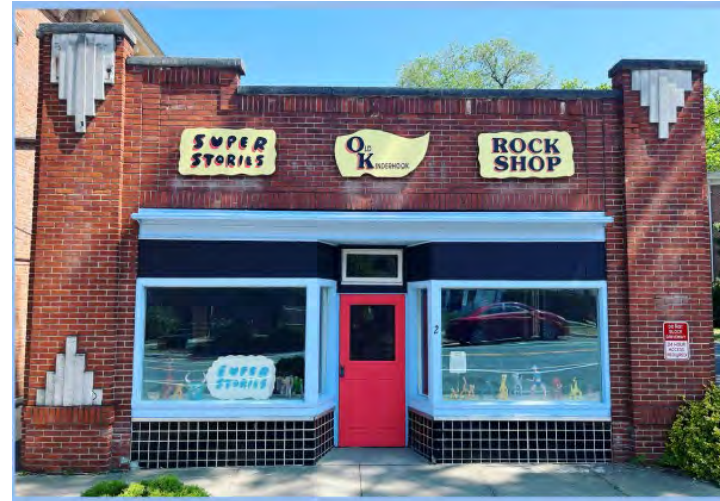
Completed work to the façade
